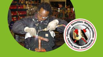
HVAC/refrigeration fitters install, maintain and service refrigeration, heating, ventilating and air conditioning systems. Marine fitters install and maintain plumbing and pipefitting on ships.
